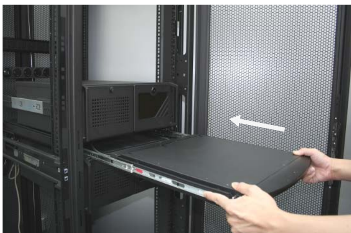
Figure 9. Pushing the LCD keyboard drawer into the rack.
